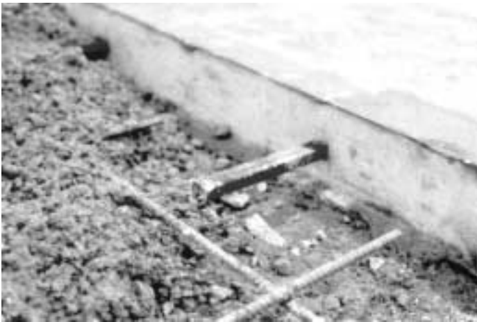
Fig. 6 – Square dowels with special clips (red) having cushioning side pads to allow differential horizontal movements but transfer vertical loads. Note: optimized concrete mixture that appears harsh and “stony” but is actually extremely workable and finishable.
