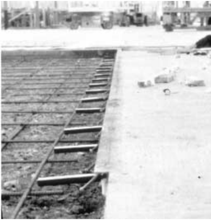
Fig. 5 – Prefabricated steel angle system for armoring floor construction joints subjected to heavy, frequent vehicle loads. For economy, armor system is located only where traffic will be. Note: square dowels with special clips (red) having cushioning side pads to allow differential horizontal movements but transfer vertical loads.
