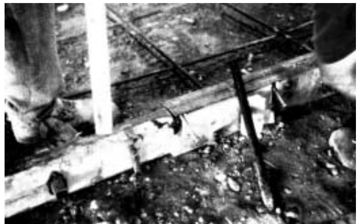
Fig. 4 – Prefabricated system consisting of steel angle armored floor construction joint, edge forms with and without armor angles, reusable dowel holders/aligners (red), etc. As adjacent slab panels shrink away from joint, elastomeric adhesive between two angles allows them to separate.
